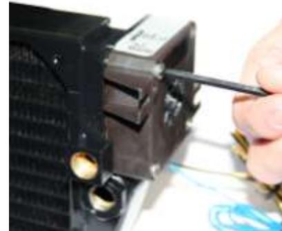
MCR220 and 320 Drive installation
